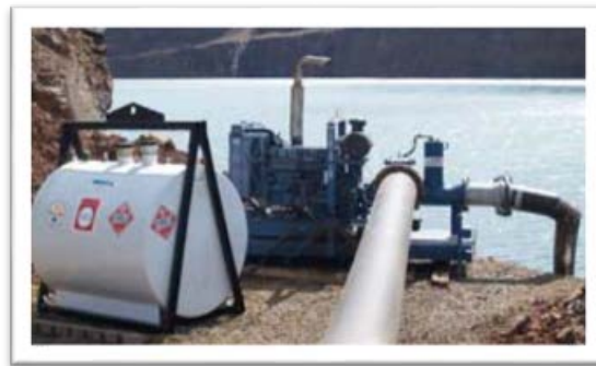
Figure 10. Dewatering mine pit in Hibbing
