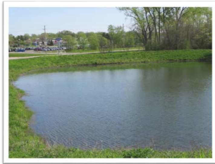
Figure 7. Large stormwater pond in Waconia will serve new commercial lots along Highway 5 as part of a regional reuse system the city will manage. Water will also be used for street sweeping.
