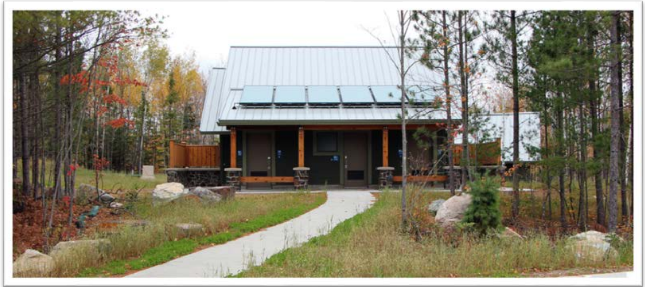
Figure 9. Shower building at Lake Vermilion State Park. Photo: SRF Consulting
