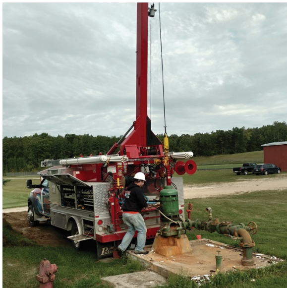
The Sebeka well sealing was one of 451 wells statewide made possible by the Source Water Protection grant program.
