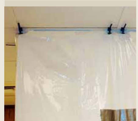
FIGURE 15 Plastic can be attached to ceiling tile grid or curtain track with clips.
