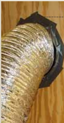
FIGURE 5 Window adapter with flex duct attached.
